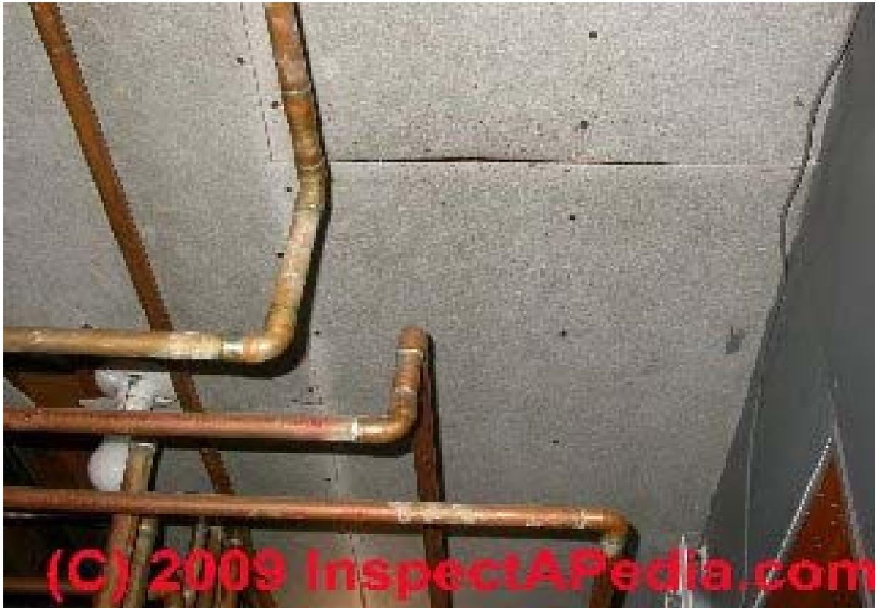
v. Paper Made of Asbestos
