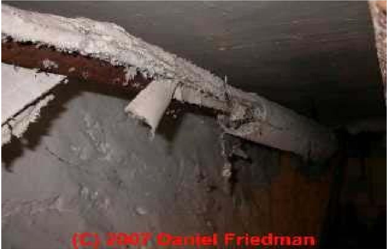
Asbestos cement pipes were used for air ducts or chimneys. Cement asbestos pipe was also used for water piping (mains in streets) and for plumbing vents on homes (photo below).
