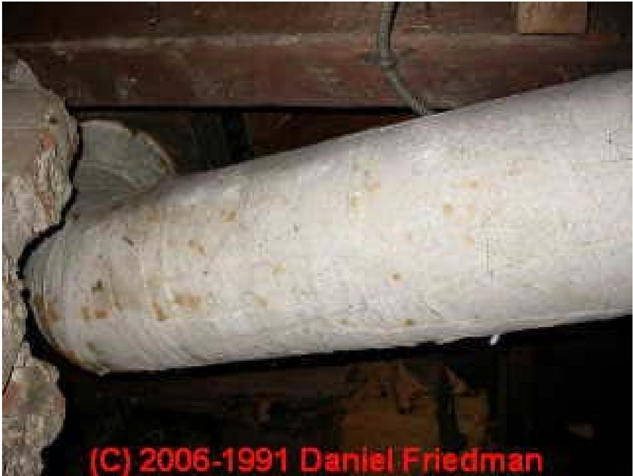
Made of high asbestos content papers (for straight pipe runs) and mastics (for pipe elbows) this insulation was applied on hot water and steam heating systems and occasionally on ordinary building plumbing piping.
