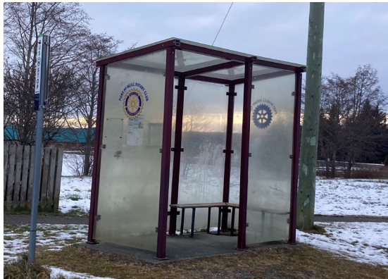
Transit Bus Shelter at Sunset Elementary School, 2025
